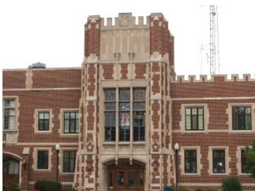
The Historic City Hall hosts one of the main Wi-Fi towers.
